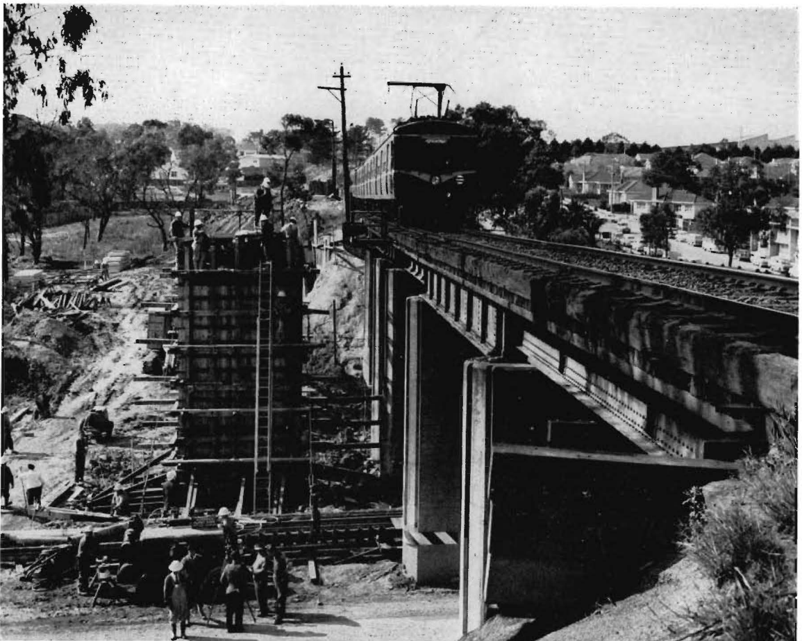
Bridge duplication work at Sydal, on the Glen Waverley line.
